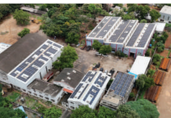
545kW - KGR Industries, Secunderabad
