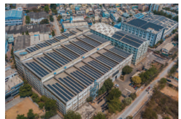
1.4MW - MTAR, Hyderabad
